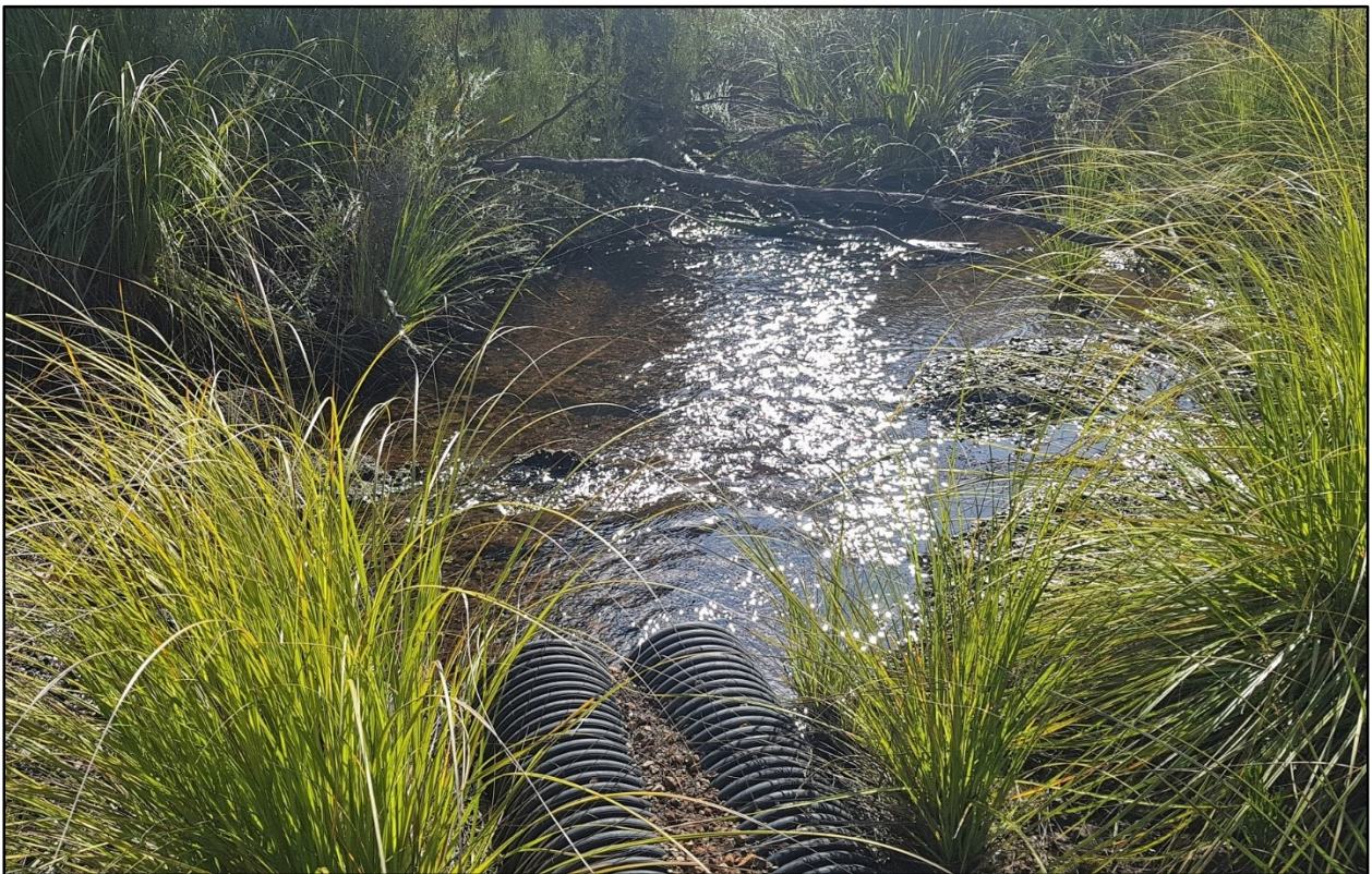
Photo 7: Several culverts have been installed on the 4WD access track where it traverses the waterway. Facing North, M.Rose, 29/08/22.
